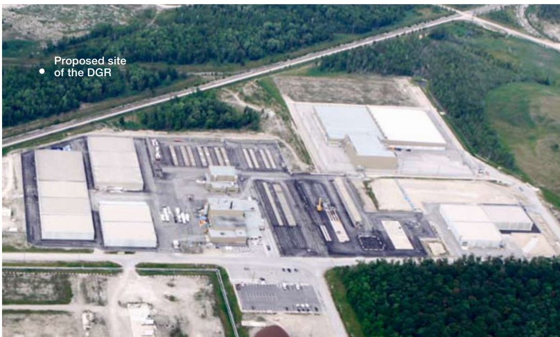
Aerial view of OPG's Western Waste Management Facility
