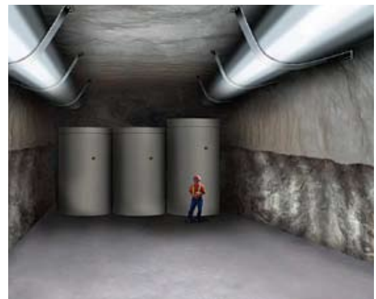
Intermediate level waste emplacement room
