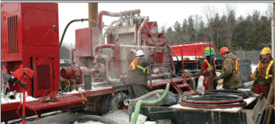
Phase one of the geoscientific site characterization activities for the Deep Geologic Repository have begun at the Bruce site. Drilling and coring of the first bore hole, which will go down to 450 metres is currently underway. The silt shaker removes particles from drilling fluid used in the process.
