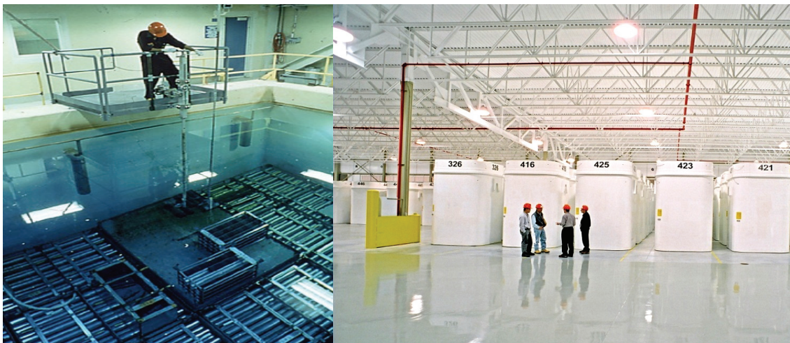
Figure 2: Example of Wet and Dry Storage of Used Fuel at Nuclear Reactor Sites
