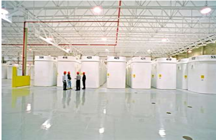
Dry Storage Containers at Western Waste Management Facility
