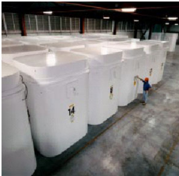
Figure 9 – Dry Storage Canisters at the Pickering Site
