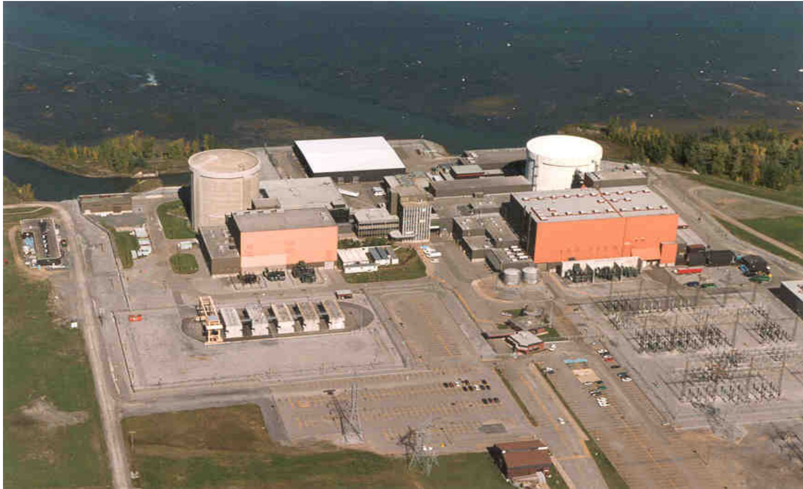
Figure 4. Gentilly Site Looking North.
