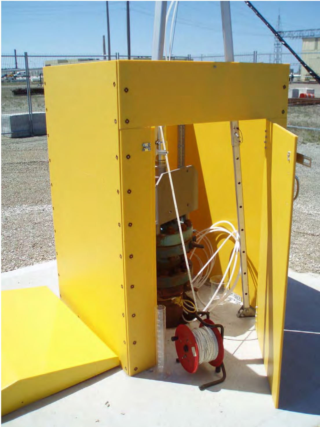
Figure 4: Example of Well Head Enclosure and Temporary Test Equipment
