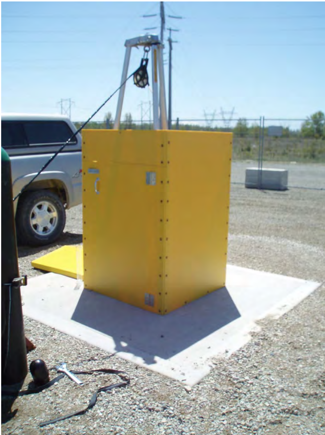
Figure 3: Example of Concrete Pad with Well Head Enclosure and Temporary Test Equipment
