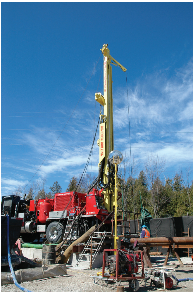
Example of rotary drilling
