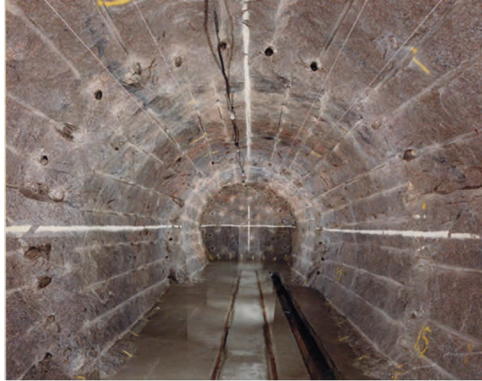
Figure 21: Long Blast Round
