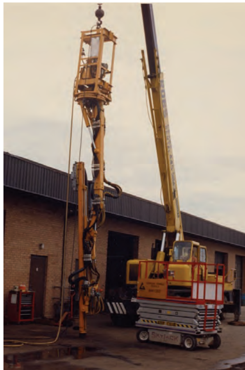
Figure 9: One of Two Drill Jumbos Used in Shaft Excavation
