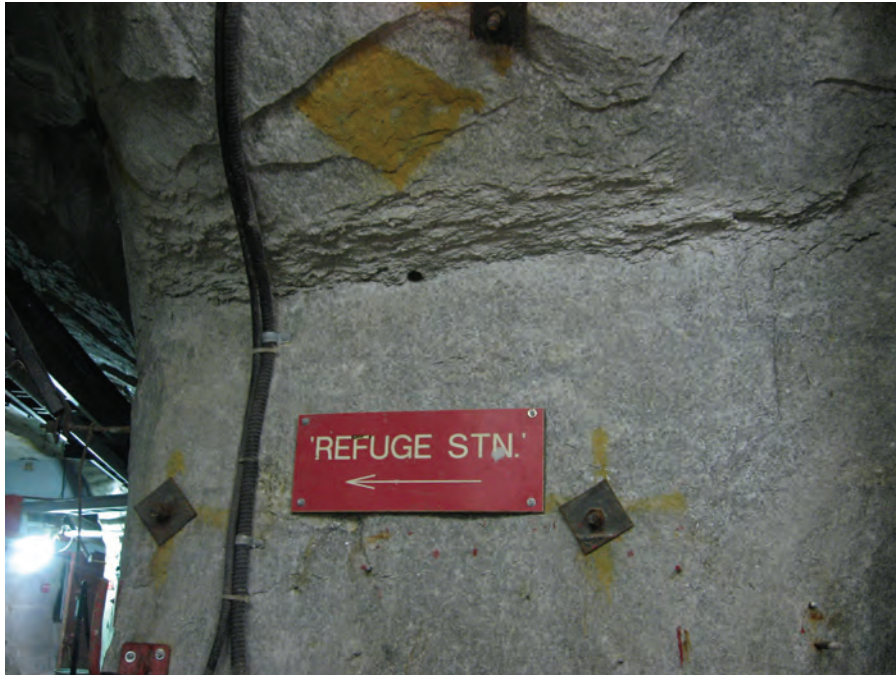
Figure 24: Stress Induced Damage at Inner Corner of Room 201
