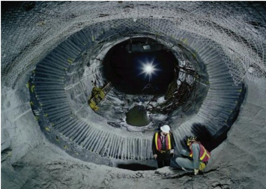
**Figure 3.2: Example of an engineering test in Canada. This photo shows excavation of the rock for a full-scale test of access tunnel seal technology at AECL's Underground Research Laboratory (Dixon et al. 2004).**
