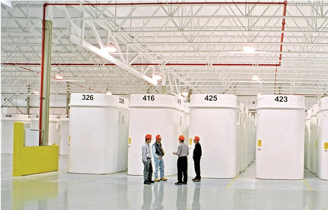
**Figure 2.2: Dry Storage Containers for used fuel at Ontario Power Generation. Each container holds 384 used fuel bundles.**
