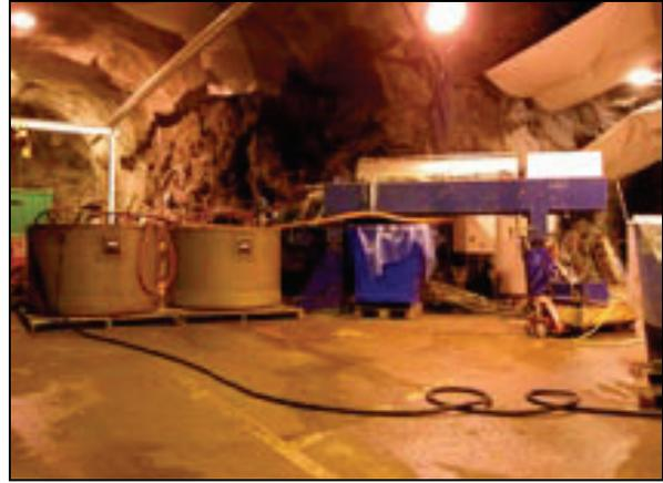
**Figure 8: Dewatering of Bentonite Slurry (SKB 2010)**
