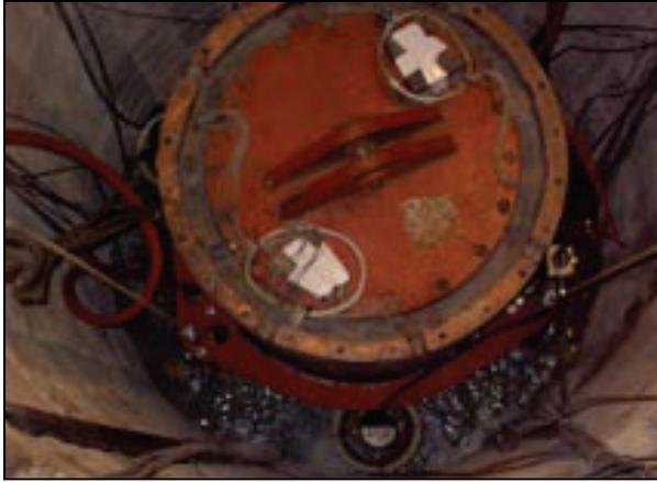
**Figure 7: Slurrying of Bentonite Buffer (SKB 2010)**
