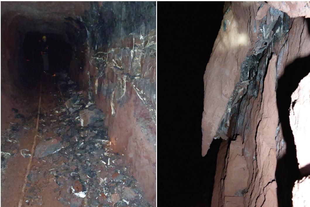
**Figure 4.5: (a) Excavation Damage (spalling) of Quintner Limestones, (b) Close up of (a)**
