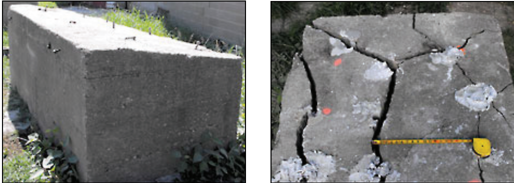
Figure 8: Use of expansive demolition agent in concrete.
