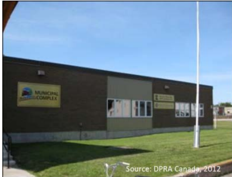
Figure 29: Schreiber Municipal Office Building
