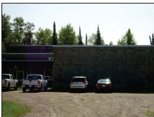
Water Treatment Plant
