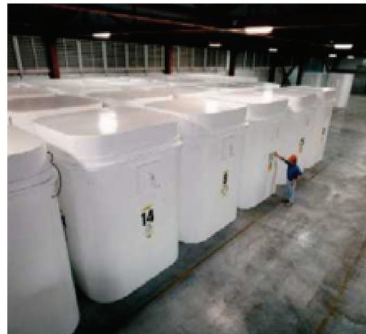
Initially, used fuel is removed from the reactor and placed in wet storage bays at the reactor site (see Figure 6-2). After a period of about seven to 10 years out-of-reactor, used fuel can be placed in dry storage at the reactor site, as illustrated in Figures 6-3 and 6-4. The long-term management approach builds on the current dry storage technology at the reactor sites.
