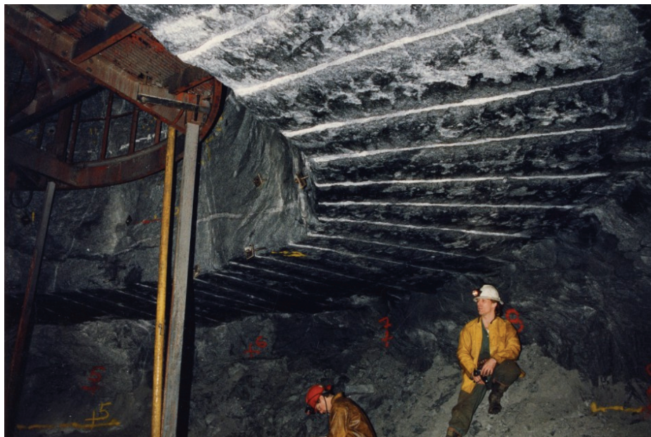
Figure 3.5: Controlled drilling and blasting used to provide smooth rock surface for geological mapping during excavation of AECL's URL
