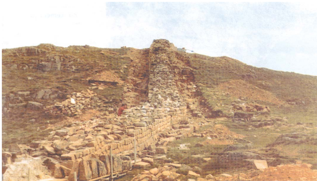
FIGURE 4 shows a present day view of Hadrian's wall showing how the overall general structure of the wall has survived for close to two thousand years (from Miller et al. , 2000, reproduced with permission from Elsevier Science).
