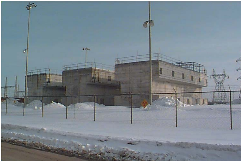
Figure 7: CANSTOR Facility at the Gentilly-2 site [46]
