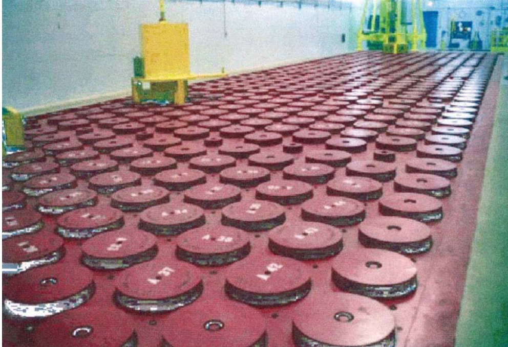
Figure 5: Example of a vault concept: Fort St. Vrain Facility in the US [34].
