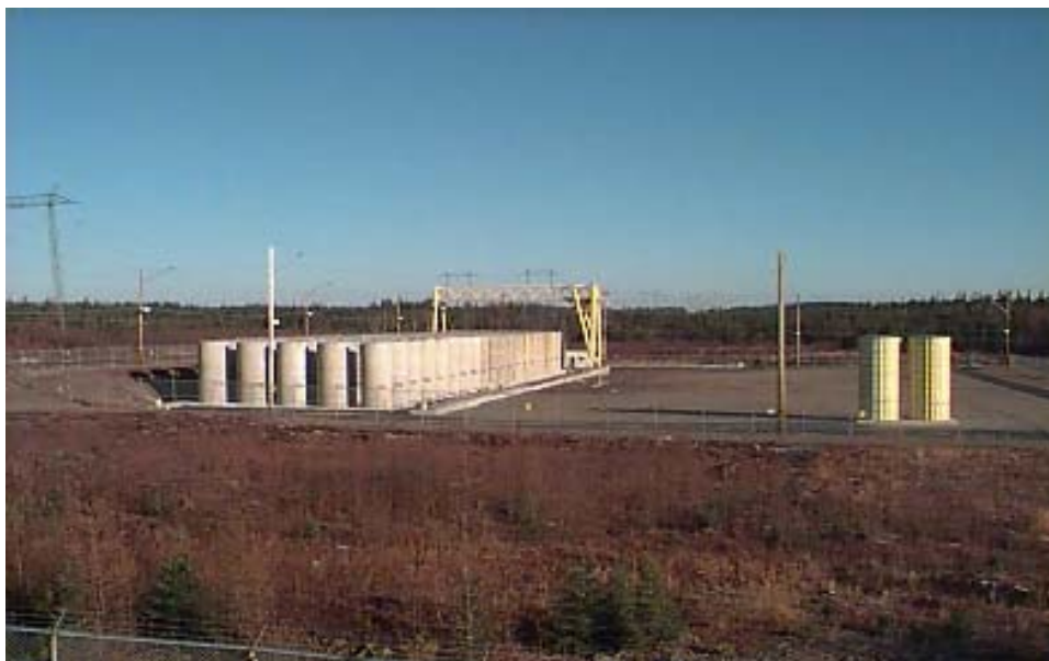
Figure 8: AECL Concrete Containers at Point Lepreau [46]
