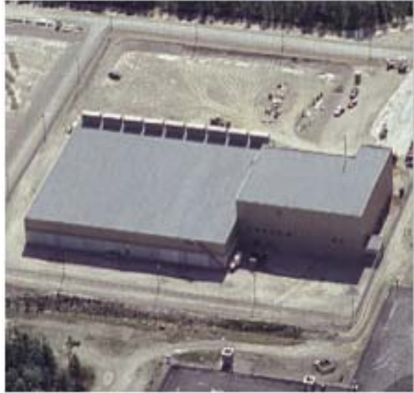
Figure 5: Example of Existing Used Fuel Storage in Dry Storage at Nuclear Reactor Sites – Surface Storage Building
