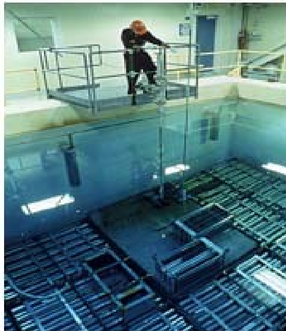
Figure 4: Example of Existing Used Fuel Storage in Wet Fuel Bays at Nuclear Reactor Sites
