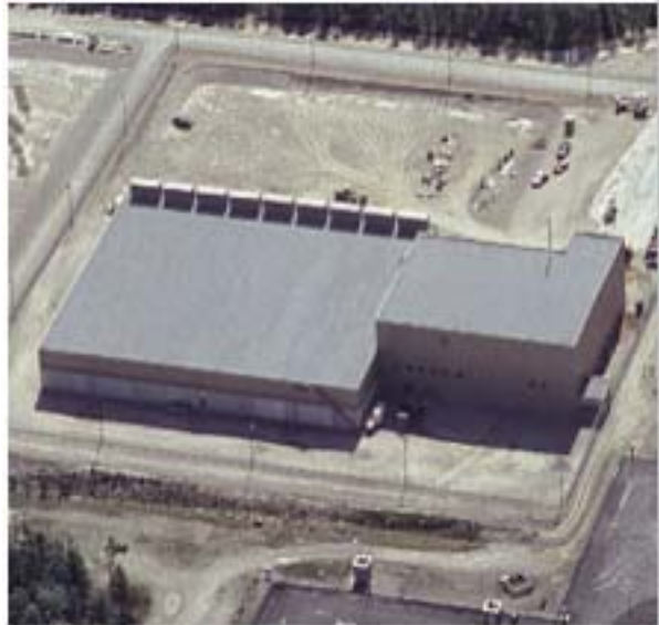
Figure 5: Example of Existing Used Fuel Storage in Dry Storage at Nuclear Reactor Sites – Surface Storage Building
