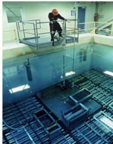
Figure 4: Example of Existing Used Fuel Storage in Wet Fuel Bays at Nuclear Reactor Sites
