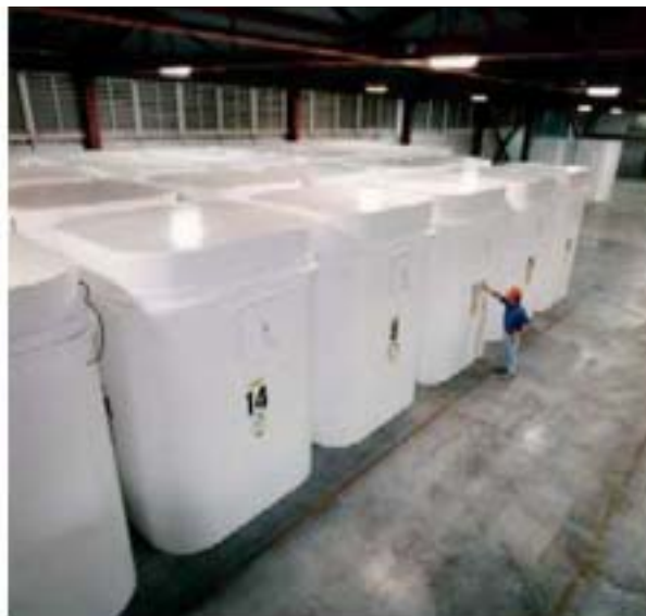
Figure 6: Example of Existing Used Fuel Storage in Dry Storage at Nuclear Reactor Sites – Dry Storage Container
