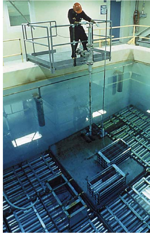
Figure 4. Spent fuel storage pool (OPG).
