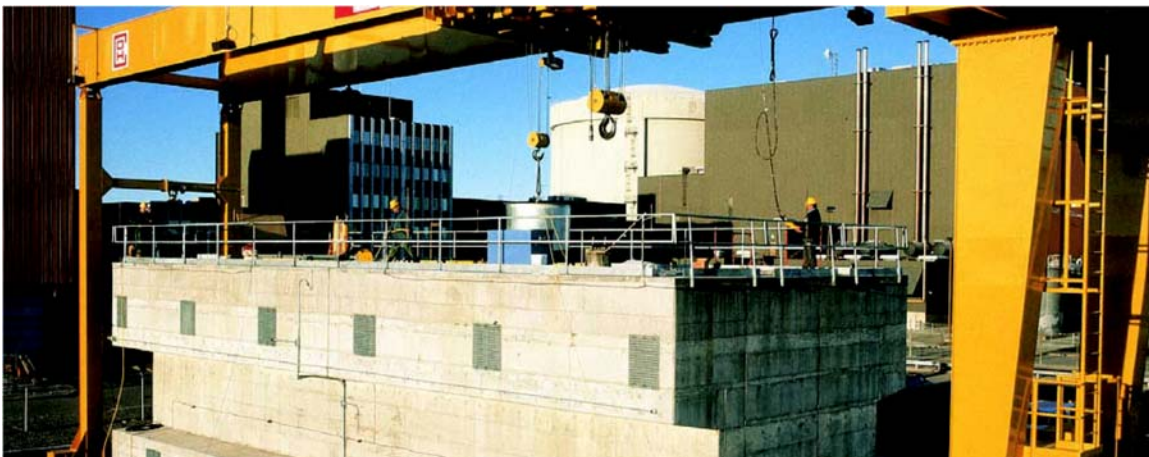
Figure D-3. Shielded transfer cask holding spent fuel is lowered into MACSTOR unit (AECL).
