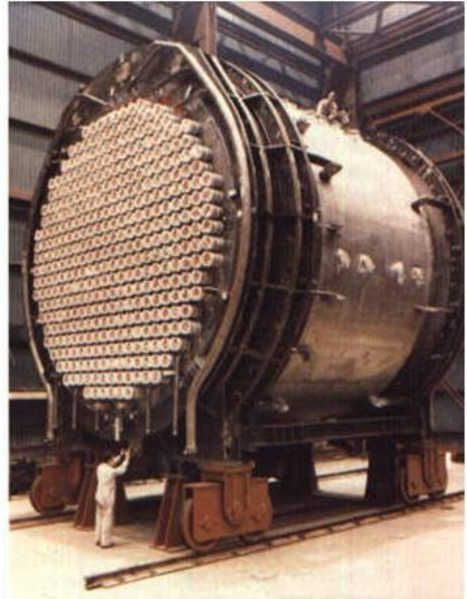
Nuclear reactor being installed
