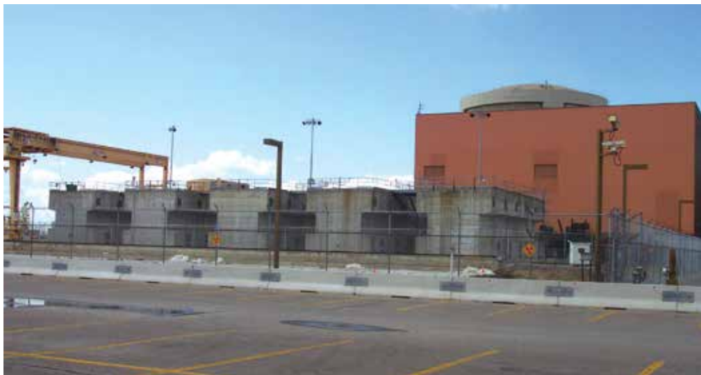
Gentilly-2 dry storage vaults
