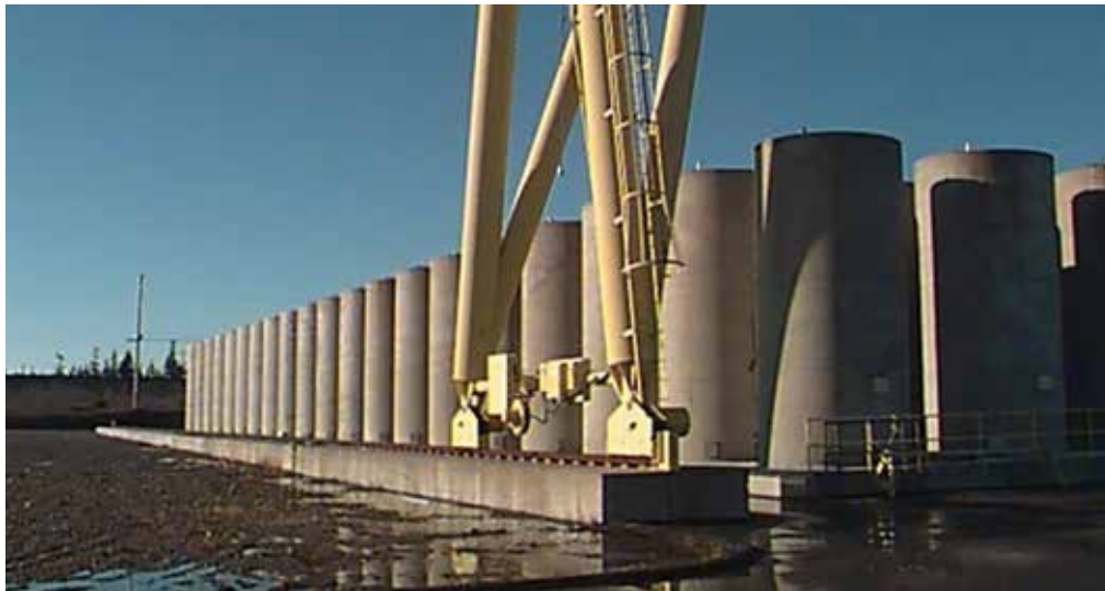
Point Lepreau dry storage silos
