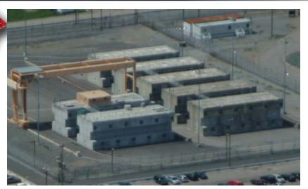
Concrete used nuclear fuel storage structures
