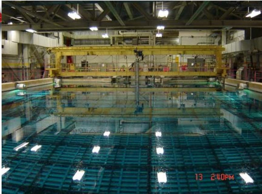
Used nuclear fuel in wet storage within reactor bays
