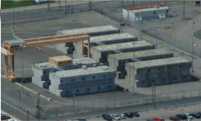
Concrete used nuclear fuel storage structures
