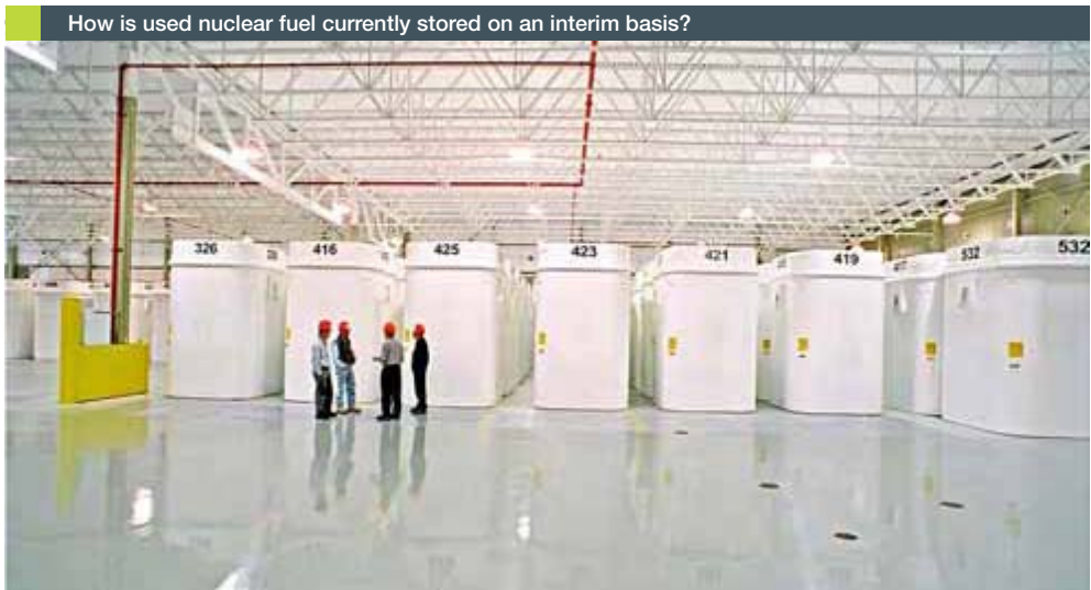
Used nuclear fuel dry storage containers at Ontario Power Generation's Western Waste Management Facility
