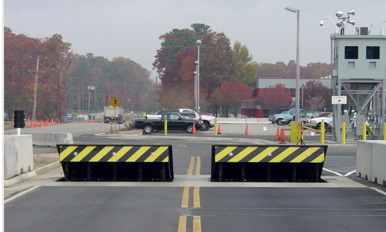
Figure 60: Vehicle Entry Point
