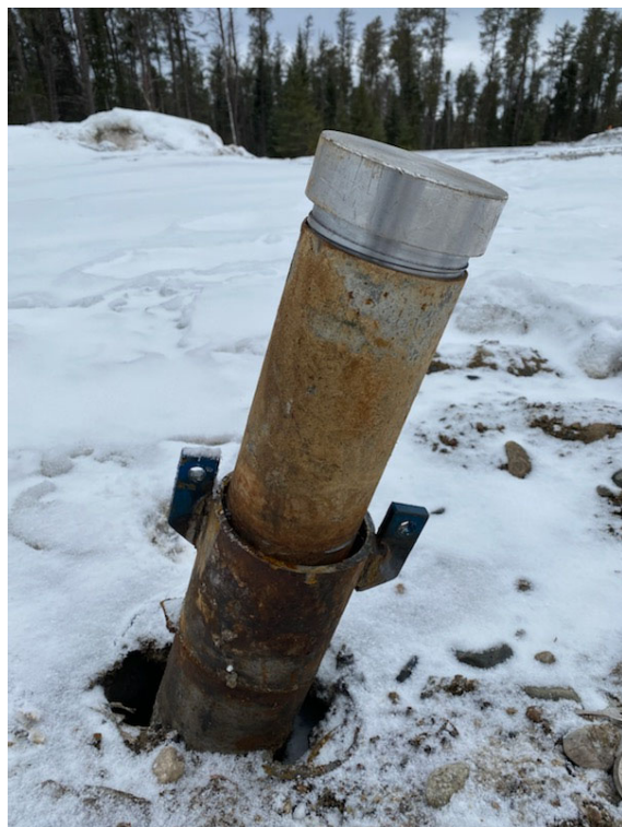
Photo 1: Aluminum plug threaded into PQT Casing, and lockable tabs welded onto PWT casing.
