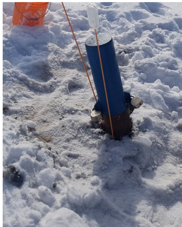
Photo 2: Lockable lid installed onto PWT Casing. With Temporary reflectors installed to prevent inadvertent contact.
