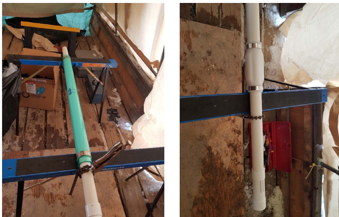
Figure 4: Photo of packer assembly on left, and abrasion protector on right. Abrasion protectors were installed directly above and below each packer, to prevent damages during assembly.
