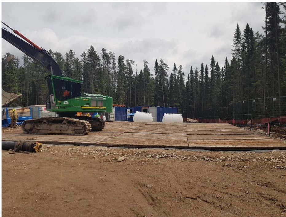
Photo 10: Facing south towards the secondary containment liner and sump used to collect spilled drill water on the drill pad. The drill pad is graded towards the central sump.
