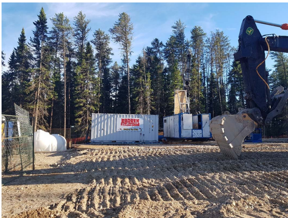
Photo 14: Facing south towards the drill rig, and core extraction shack, sitting on the drill pad secondary containment and rig matting.
