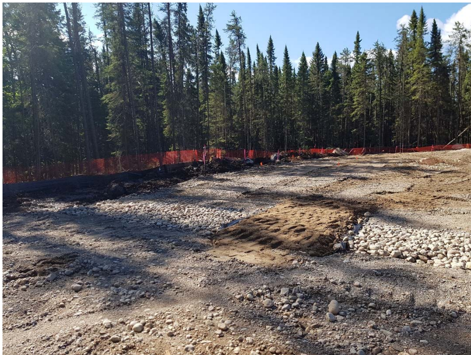
Photo 2: Facing south from the northeast corner of the drill site. To assist in self-drainage at the north end of the site, a drainage swale was dug into the subgrade, and was backfilled with cobbles to allow easterly movement of rainwater off of site. Walking paths were created next to the anticipated office trailer locations to mitigate tripping hazards associated with walking on cobbles.
