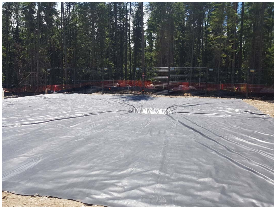
Photo 10: Facing south towards the secondary containment liner and sump used to collect spilled drill water on the drill pad. The drill pad is graded towards the central sump.
