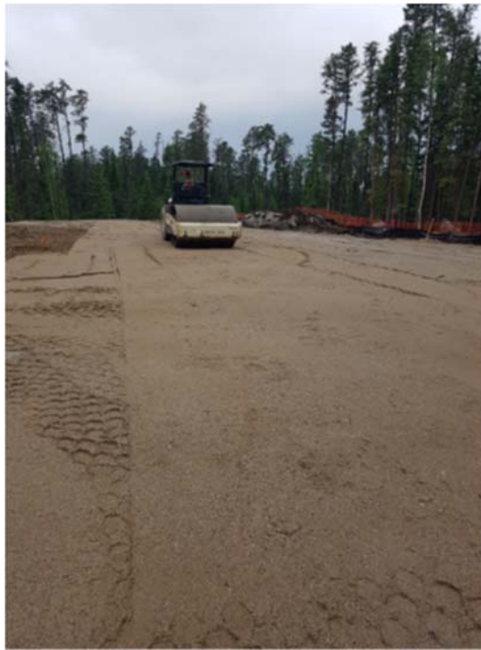
Photo 1: Facing west towards the entryway to IG_BH02. A smooth drum roller was used to compact the final lift of subgrade material at IG_BH02
