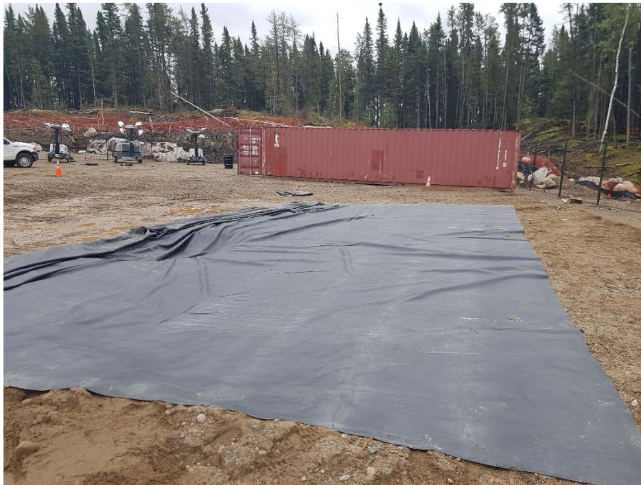
Photo 7: Facing east towards the secondary containment liner and sump used to collect spilled drill water on the drill pad. The northern half of the containment liner is rolled up so that the excavator can place rig mats without damaging the liner.
