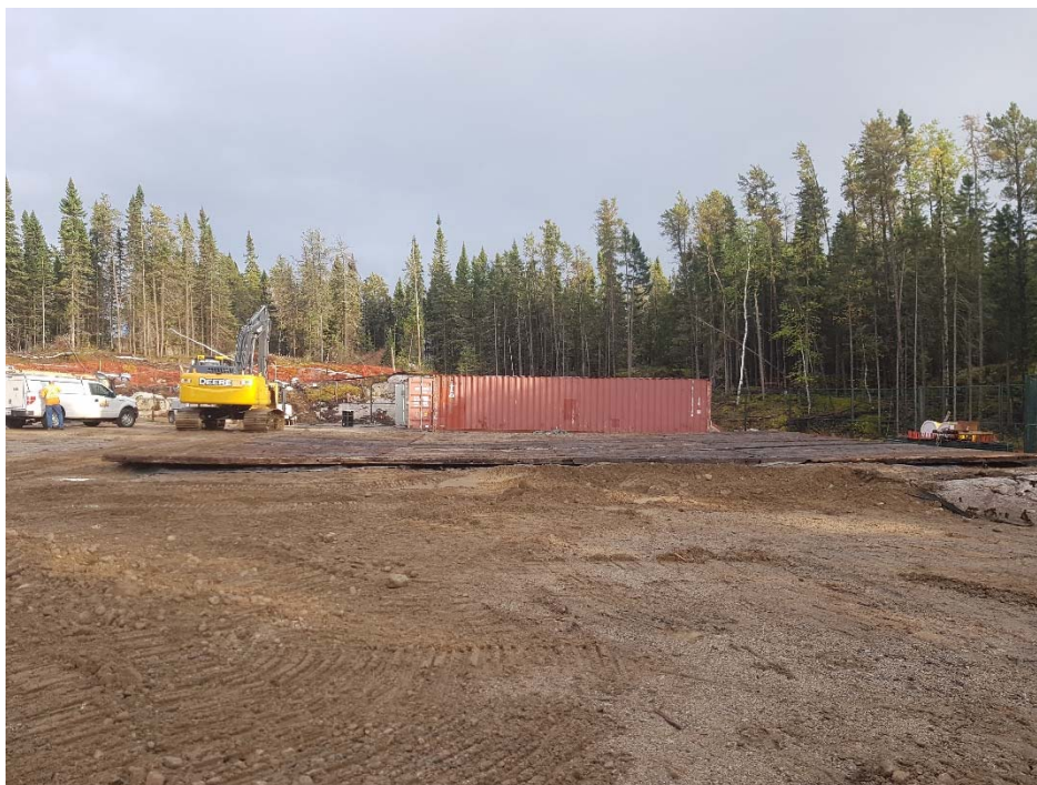
Photo 8: Facing east towards the rig matting which was placed over top of the drill pad secondary containment liner
