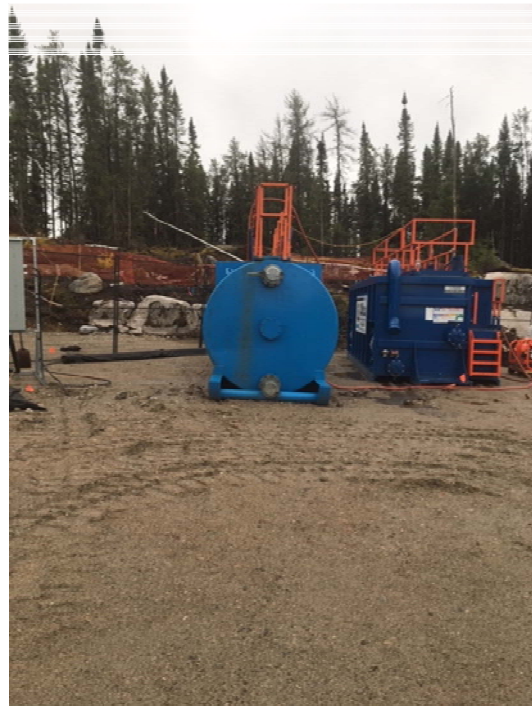
Photo 13: Facing south towards one of the two 28,350 L baker tanks located on the east side of site. The baker tanks are used to store source water supplied from the Township of Ignace.
