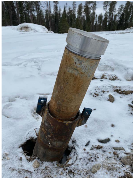
Photo 3: Facing west towards the aluminum plug fabricated to temporarily seal the top of the IG_BH02 borehole casing. The plug was installed on March 18, 2020
