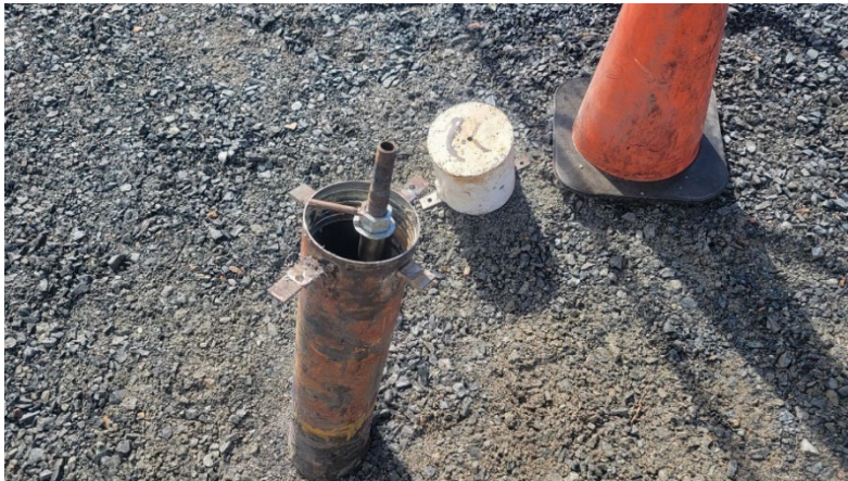
Photo 1: Lid removed to show mechanical packer installed, before painting and locking of extended casing monument.
