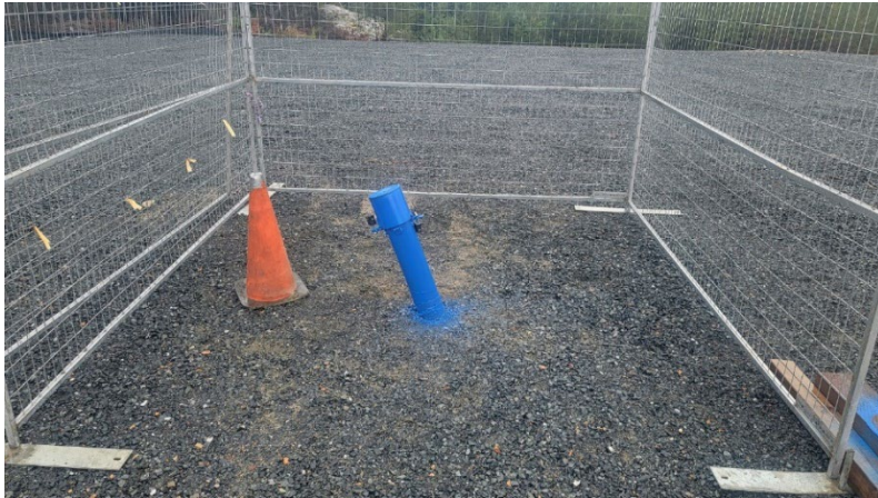
Photo 2: Lockable lid installed onto conductor casing with secondary physical barrier (cage) to prevent incidental contact.
