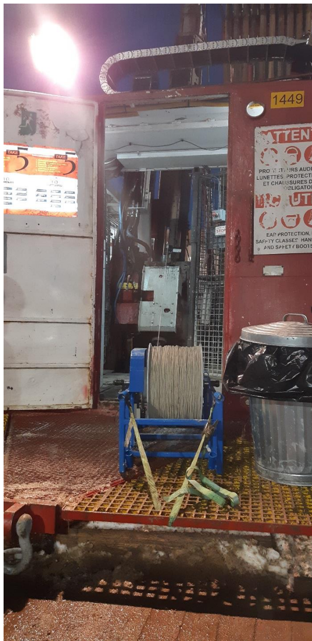
Photograph 1. Verifying passage down hole is clear of obstruction.
