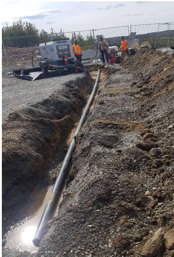
Photo 18 - Trench construction to bury the power cables.
