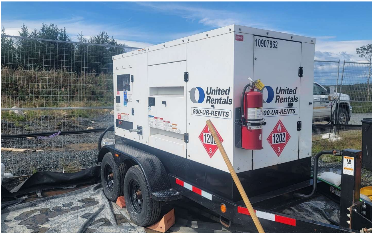
Photo 16 - Cummins mobile diesel generator (model C60D6R) in secondary containment with a fire extinguisher.
