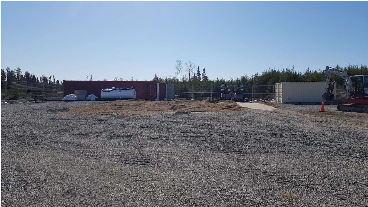
Photo 10 – Placement of the sand layer prior to the secondary containment construction.
