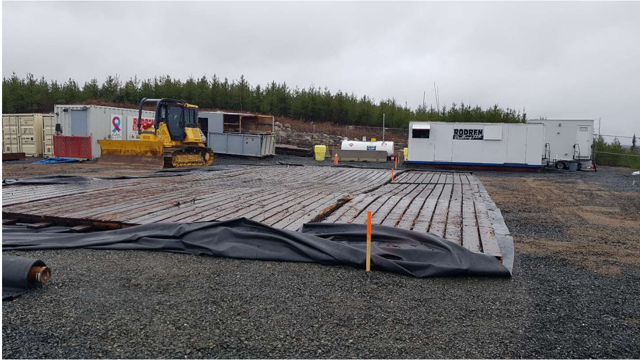
Photo 11 - Placing wooden rig mats.
