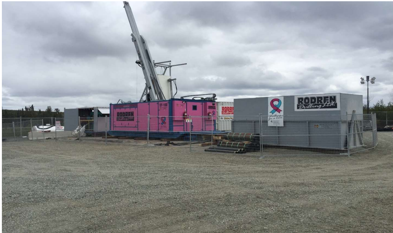
photo 3 - 1.8 m Tall drilling zone fence
