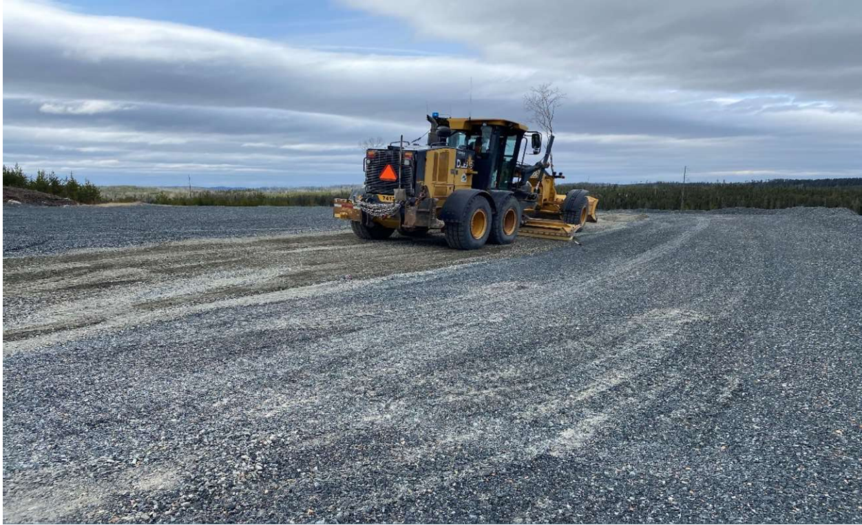
Photo 1 - Grading out the edge of the drilling pad for easy access and setup
