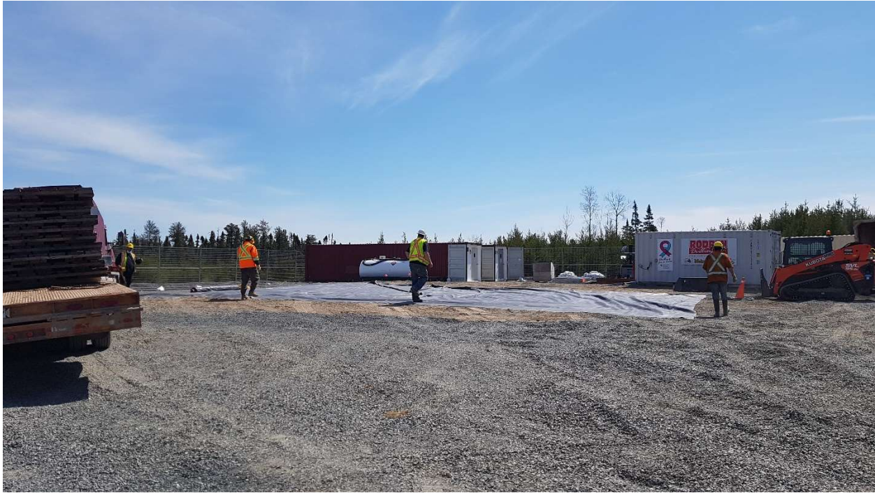
Photo 9 - Drill pad secondary containment construction.
