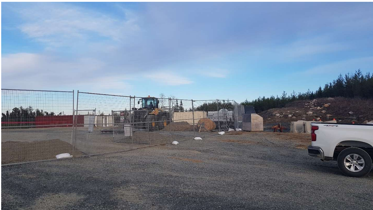
Photo 2 – 2.1 m Tall site security fence with lockable gate
