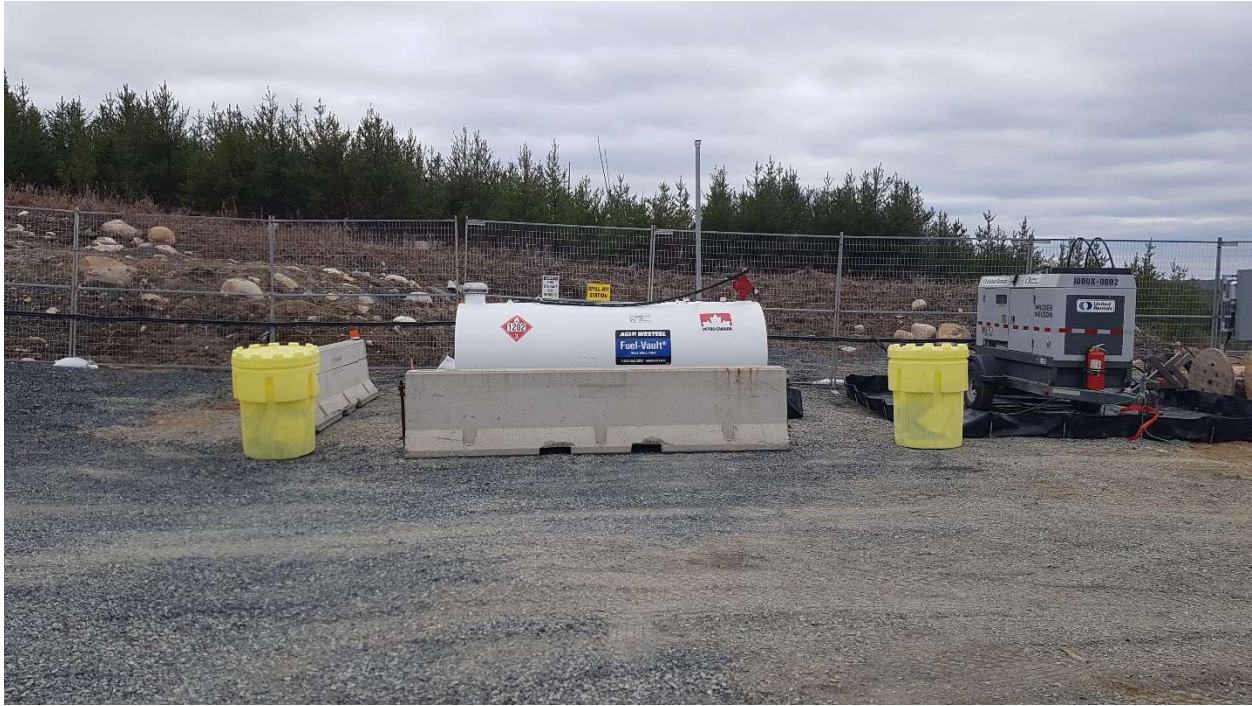
Photo 21 - Spill kits around the fuel tank.
