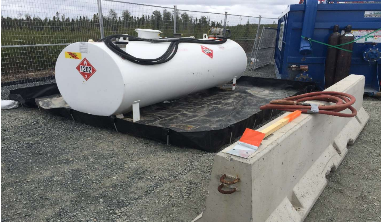
Photo 17 - Double-walled fuel tank - 4500 Litres.
