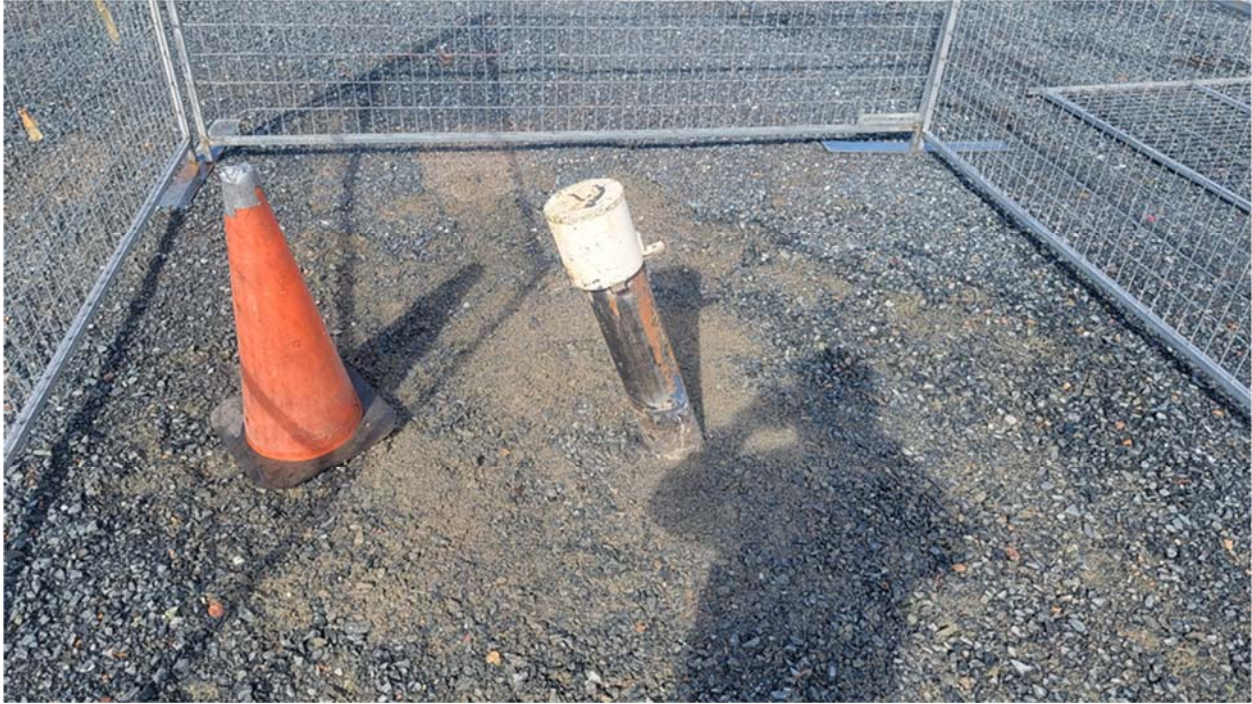
Photo 7 – IG_BH04 wellhead after restoration. A new section of outer casing was welded by Rodren and the previous casing cap was reinstalled - September 5, 2021.
