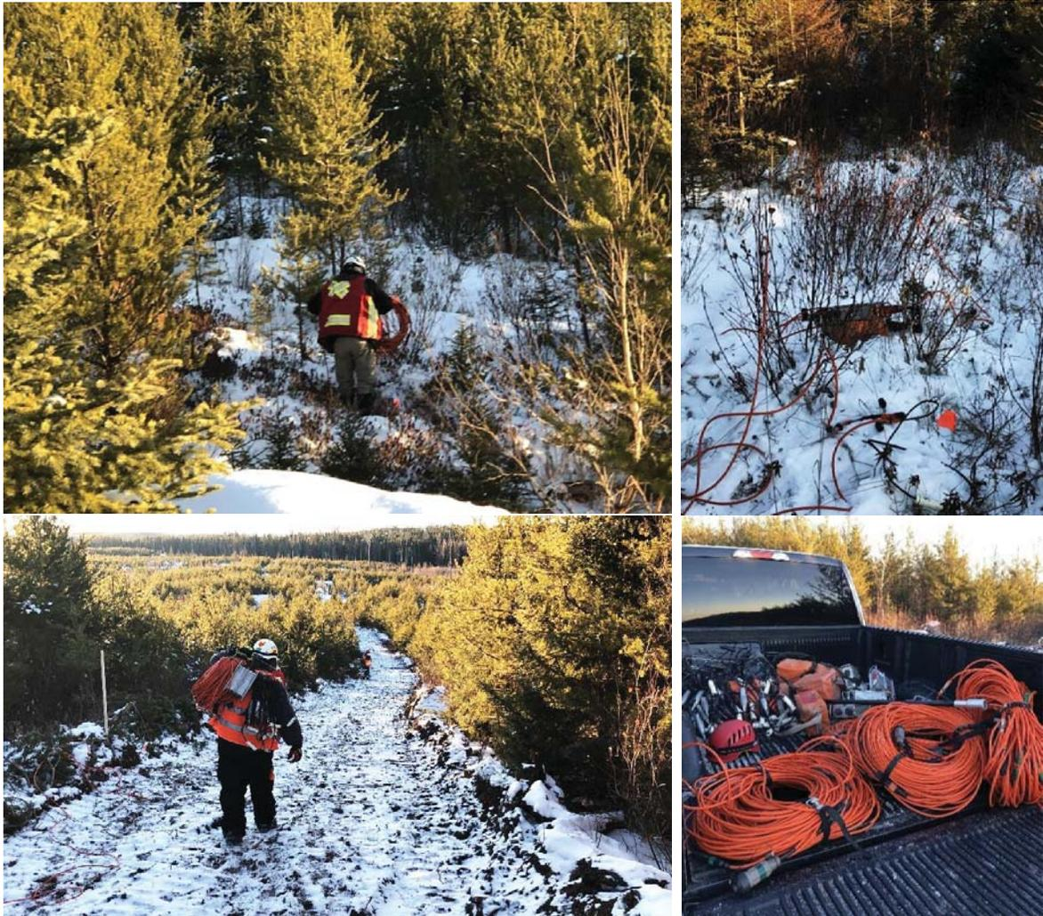
**Figure 3. Installation of the acquisition system in the field, both on the line extensions (top) and along the lines (bottom).**
