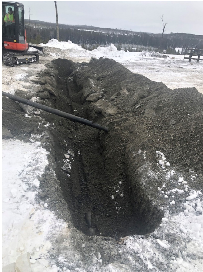
Photo 6 – Underground electrical conduit excavation and removal – November 18, 2021
