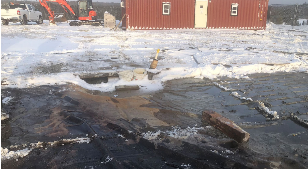
Photo 3 – Rig mats removed from IG_BH05 drill pad, secondary containment in process of being removed - November 18, 2021
