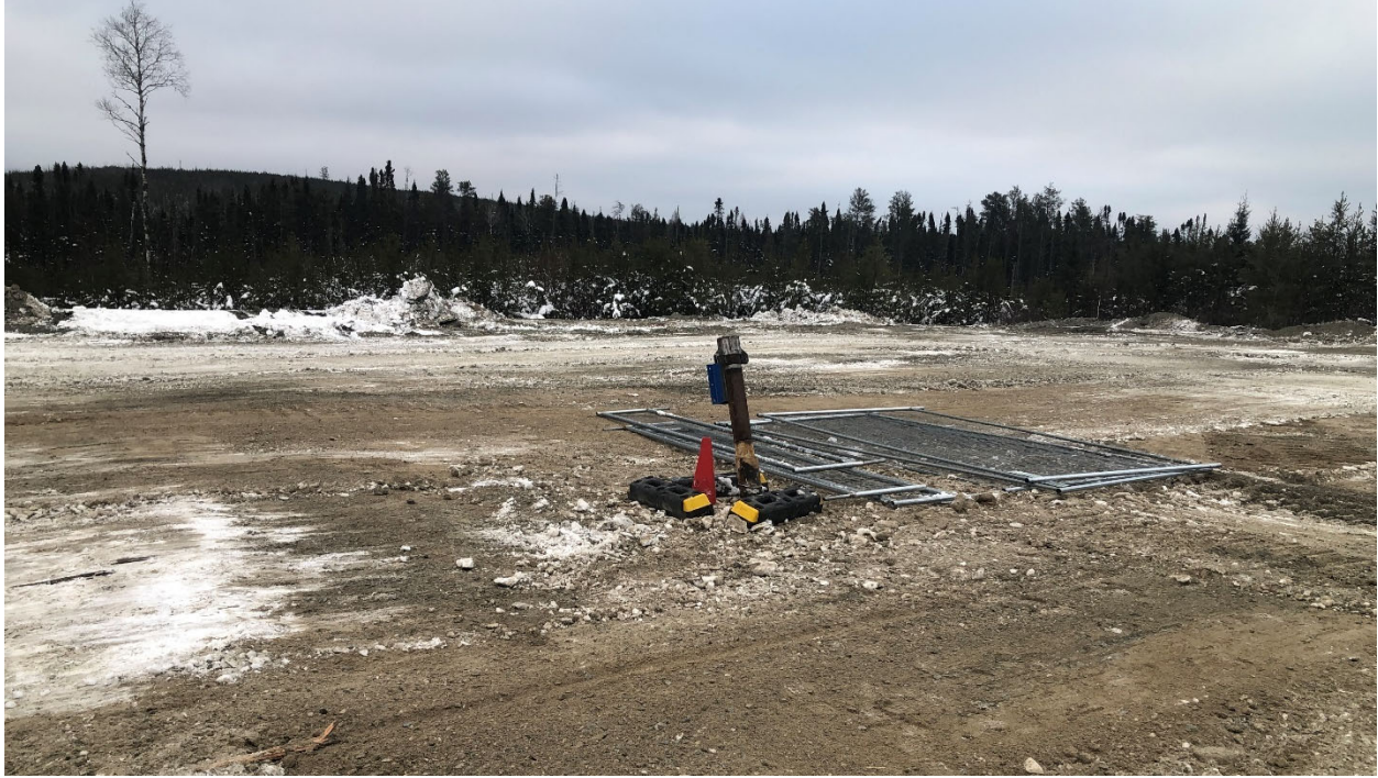
Photo 7 – Final site condition with final wellhead casing installed, NWMO supplied locks in place, grading complete - November 20, 2021
