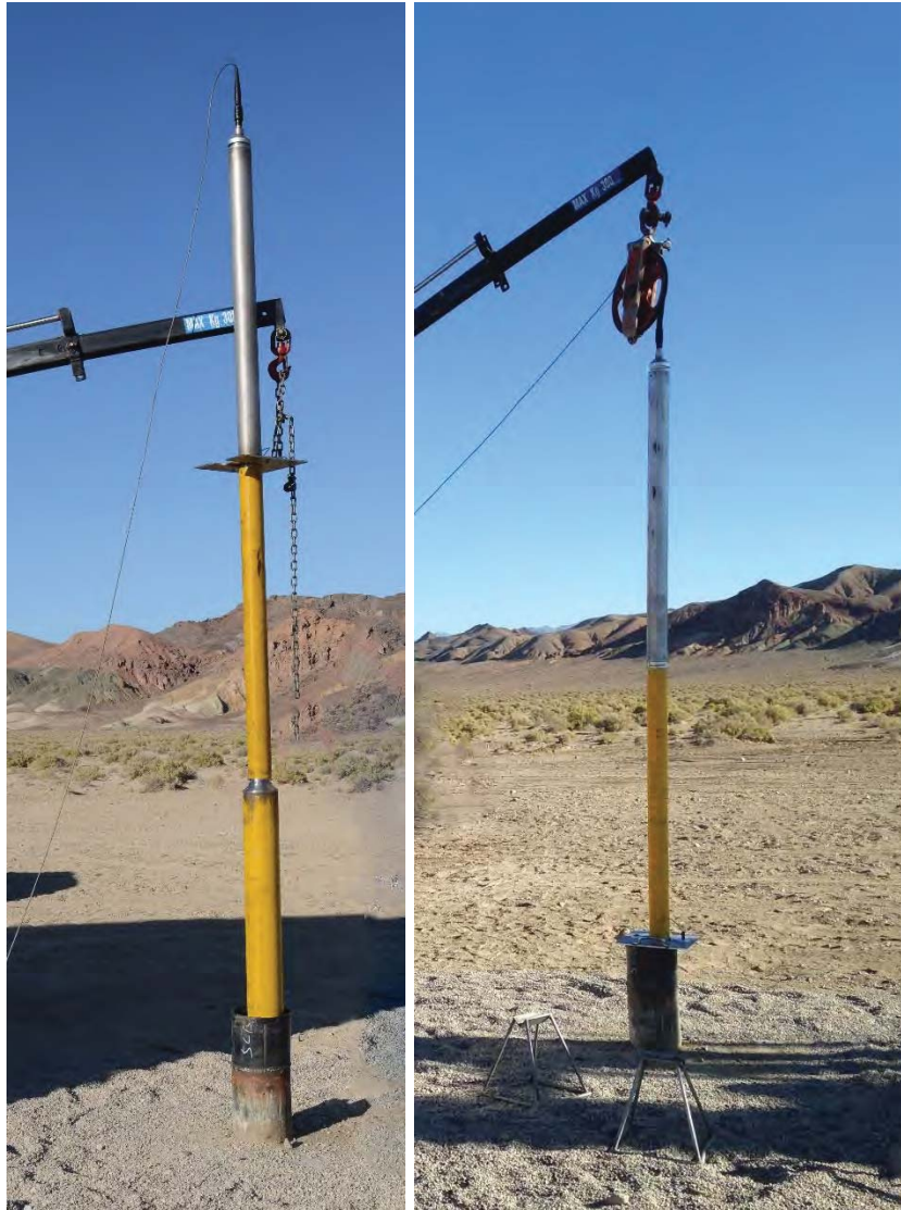
Figure 38: Lowering the tool string into a well using a landing plate/C-plate and crane (left). Transitioning the weight of the tool string to the logging cable (right).
