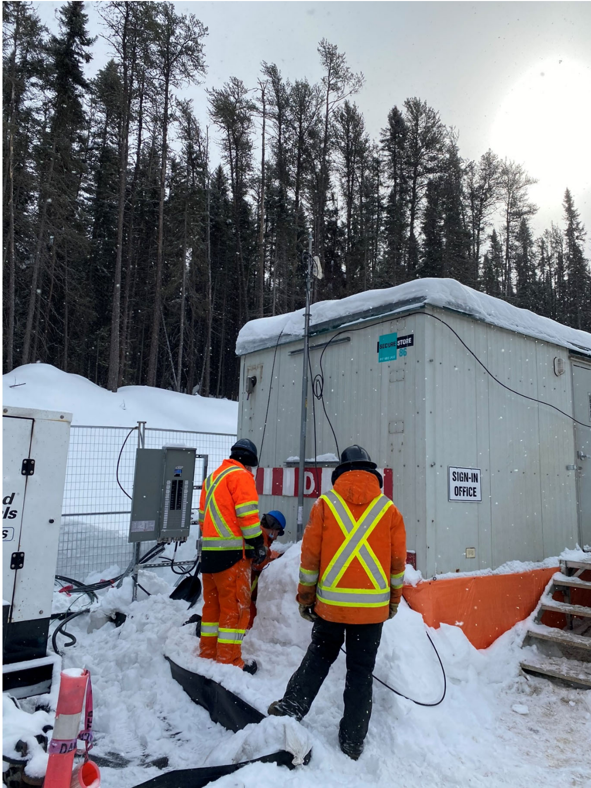
Photo 5 – Communication system disconnect & removal, taken February 28, 2022
