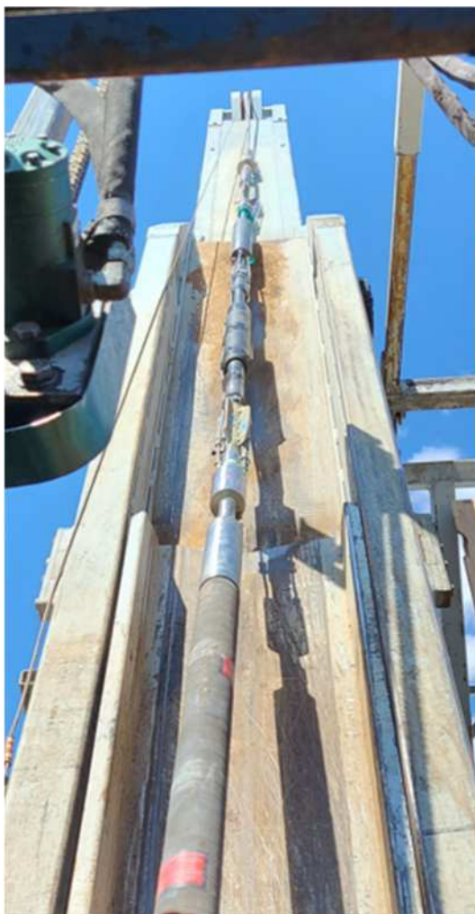
Photo 2 – Datalogger, DHSIV and upper packer shown assembled at drill rig.
