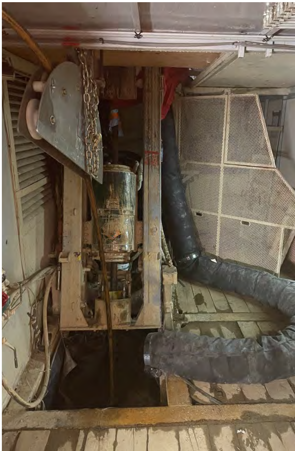
Photo 5 – Flatpack shown entering BH06 via and sheave wheel at the rig mast with temperature control (black conduit).
