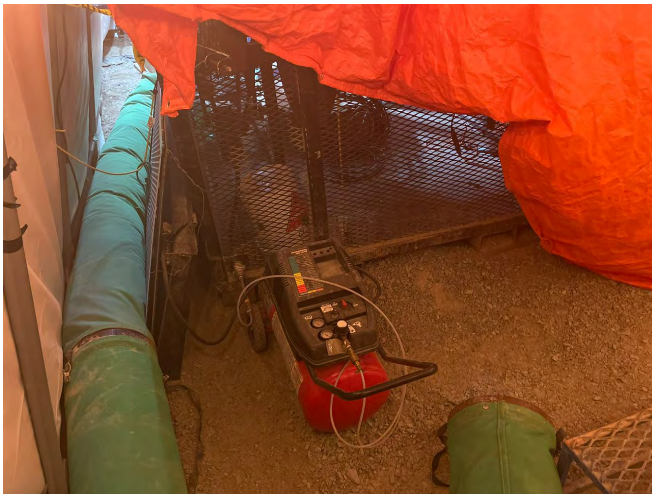
Photo 2 – Rear of flatpack cage with compressor and temperature control (orange tarps and green heating conduits).
