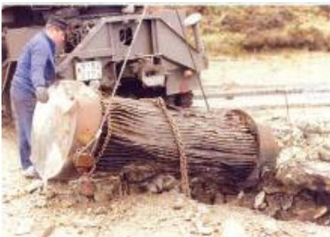
**Figure 4-10: Package after lifting off the concrete ground**
