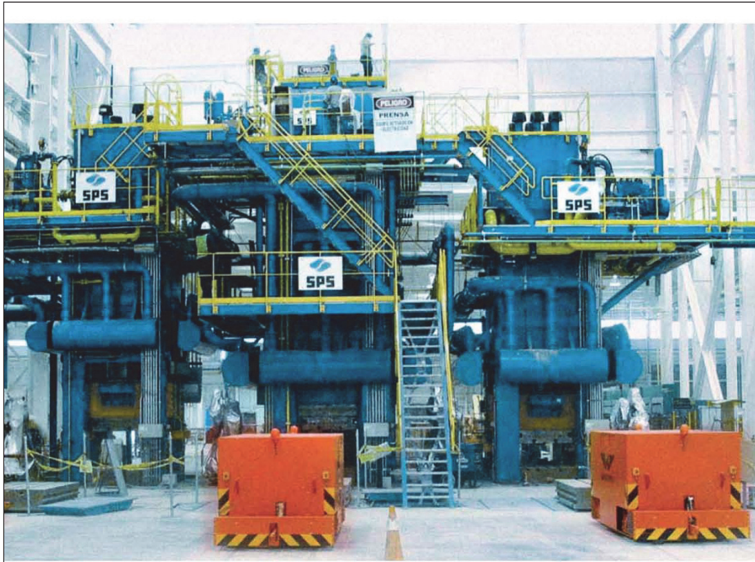
Figure 3-6: Example of a Large Press for the Sealing Material Compaction Plant
