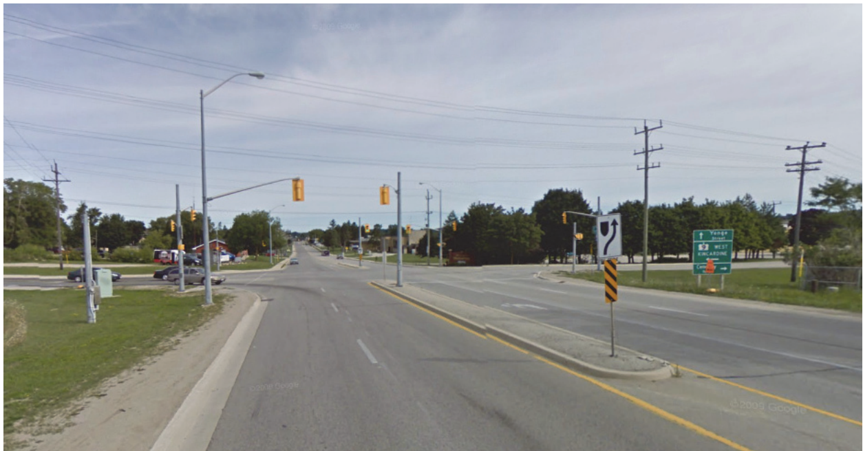
Figure 6-3: Highway 9 near Brockton (Walkerton)
