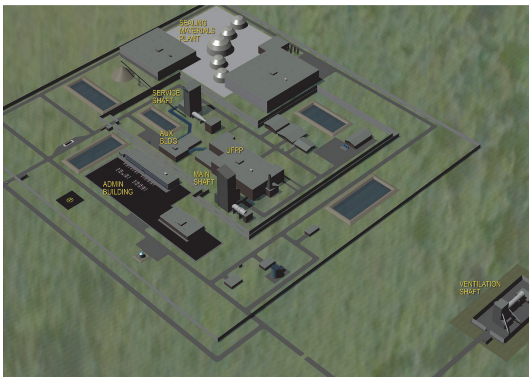
Figure 3-3: APM Surface Facilities
