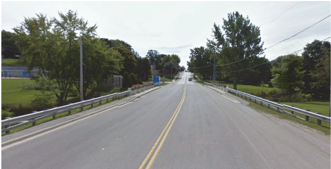
Figure 6-3: Highway 9 near Mildmay in South Bruce
