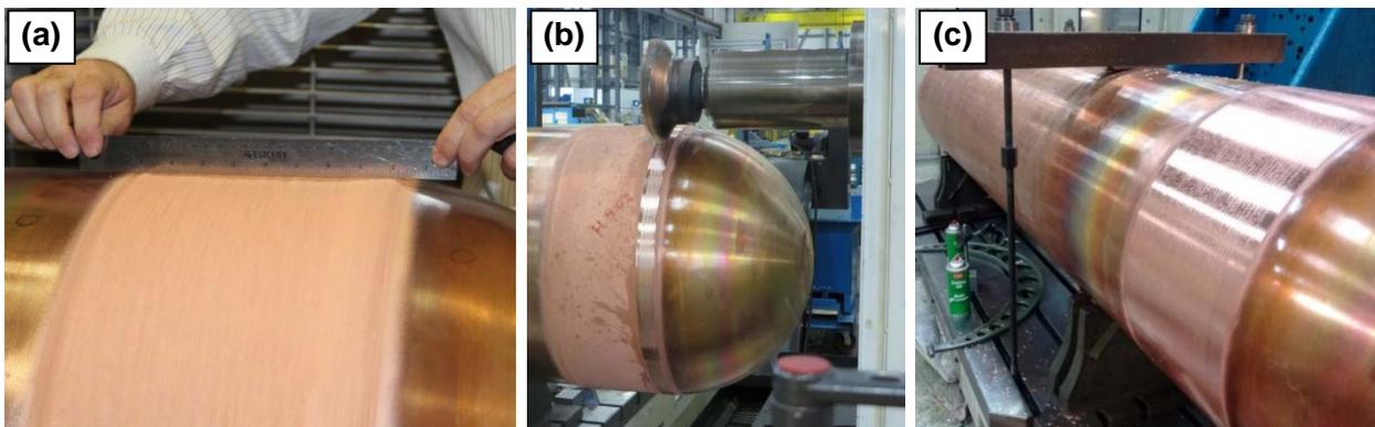
**Figure 3.17: Cold Spray Copper Coating Applied to Closure Weld Region (a) Before (b) During and (c) After Machining**
