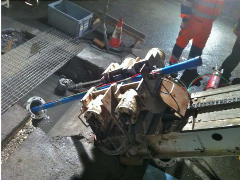
Picture 3: Artesian outflow after installation of packer but before packer inflation (Fr, 13.12.2013).
