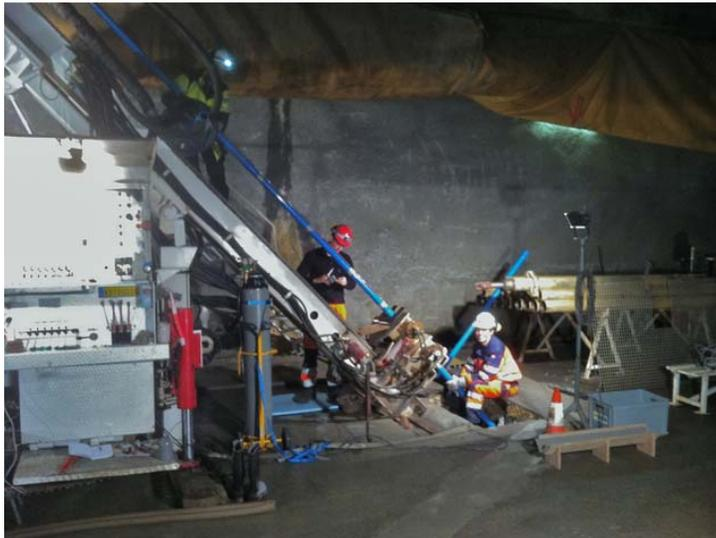
Picture 2: Installation of packer system (Fr. 13.12.2013).
